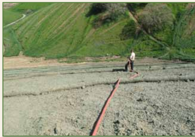
Erosion and Sediment Control
